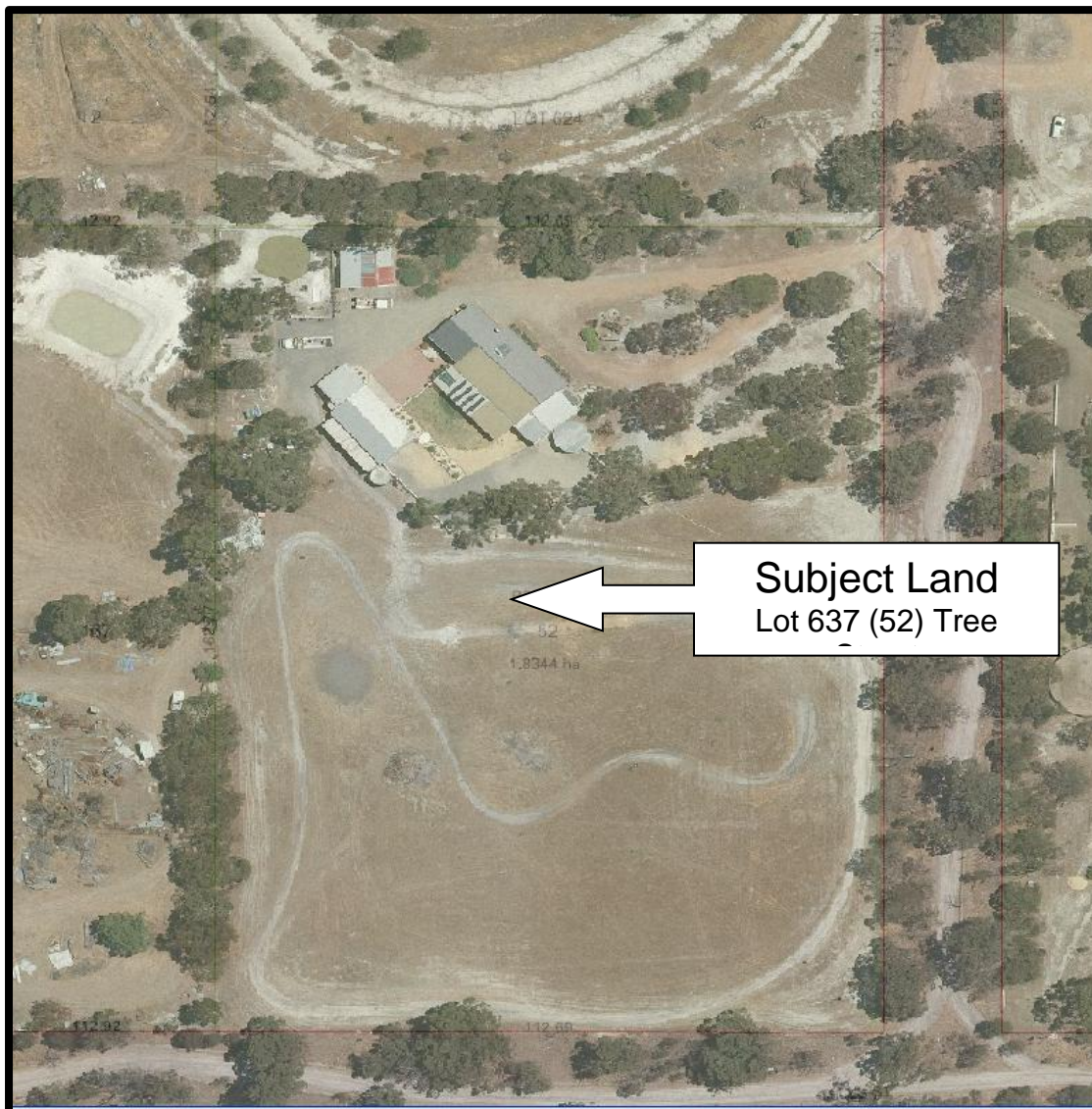
Aerial Image of Lot 63752 (52) Tree Street
