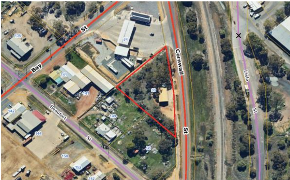
FIGURE 1 A2244, 30 CORNWALL STREET, KATANNING
