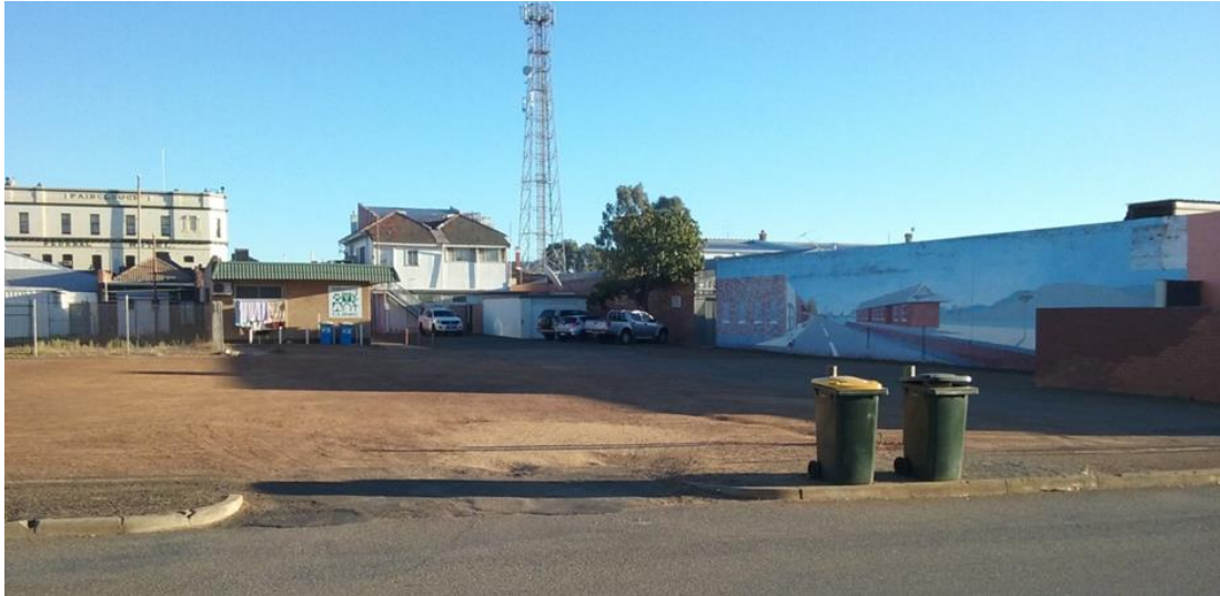
Rear view of existing premises (from Baker Street) showing crossover and parking area.
