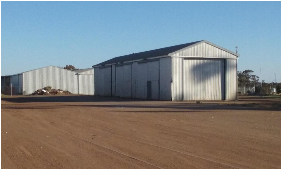
Northern elevation of vacant premises – Pt Lots 847 & 848
